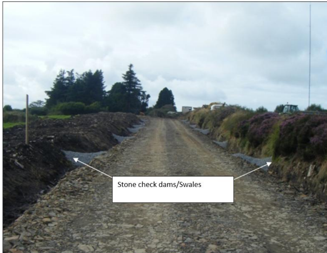
Figure 3-19: Examples of Check Dams Along Access Track Drainage Channels
