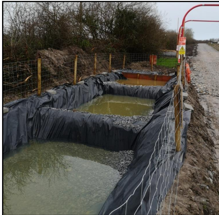
Figure 3-18: Multi-tiered Settlement Pond with Stone Filter
