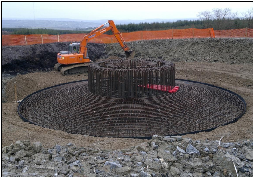
Figure 3-7: Typical Wind Turbine Base
