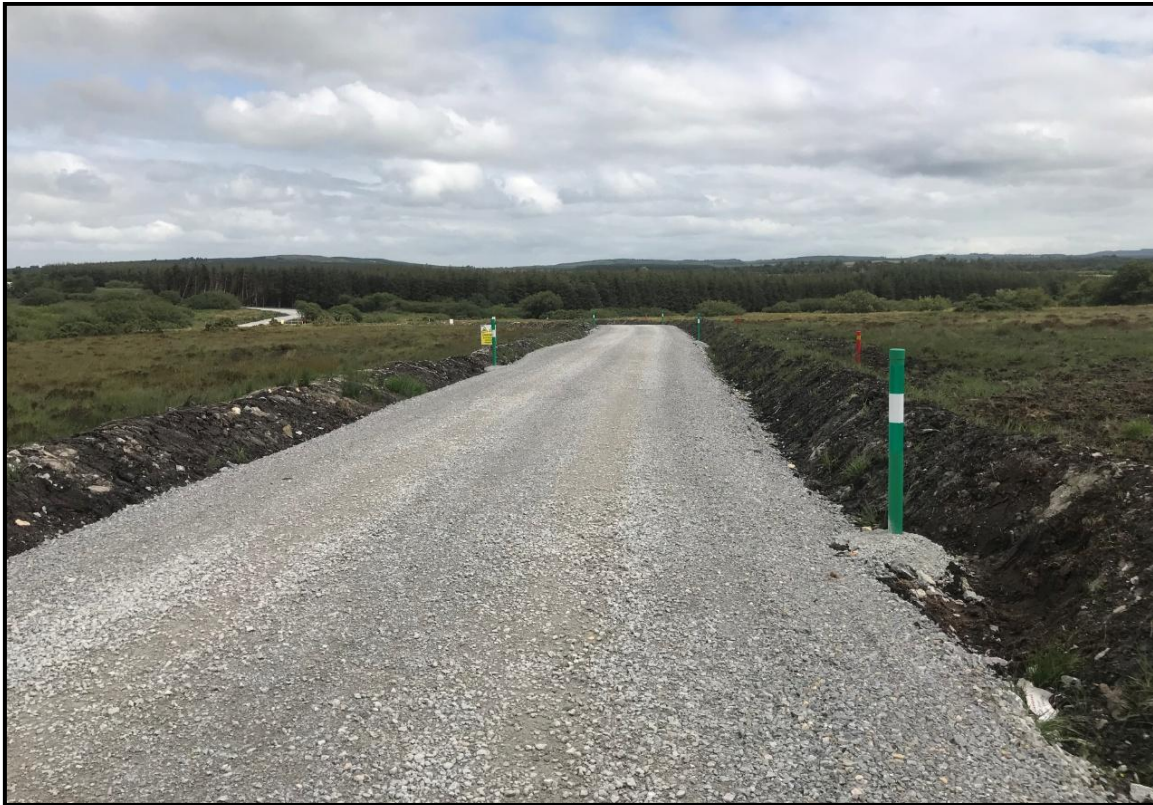
Figure 3-5: Typical Floated Track
