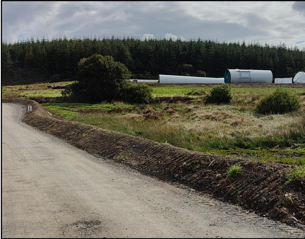
Figure 3-15: Dirty Water Containment Berm
