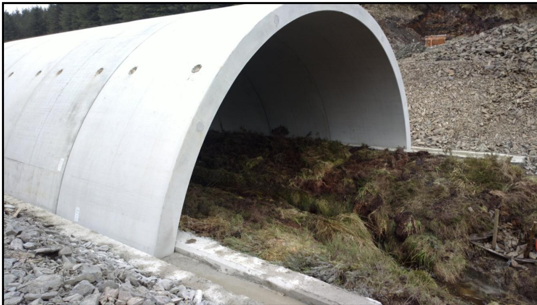
Figure 3-12: Typical Construction of a Clear Span Pre-Cast Concrete Arch Unit
