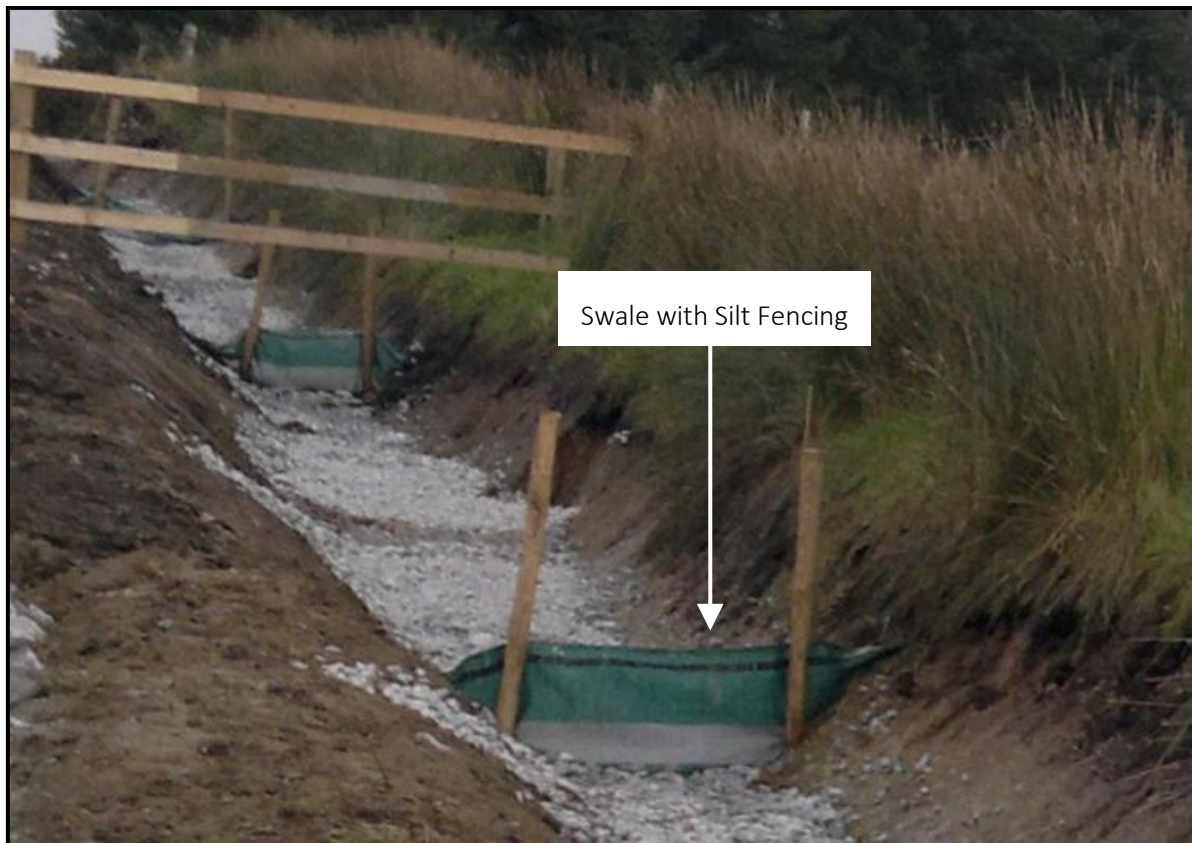
Figure 3-20: Example of a Silt Fence in a Swale
