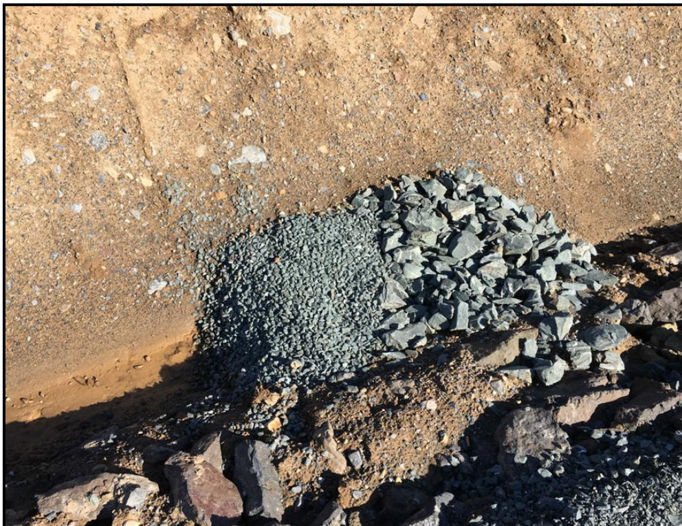
Figure 3-17: Stone Check Dam (With Large Aggregate on Downstream Side)
