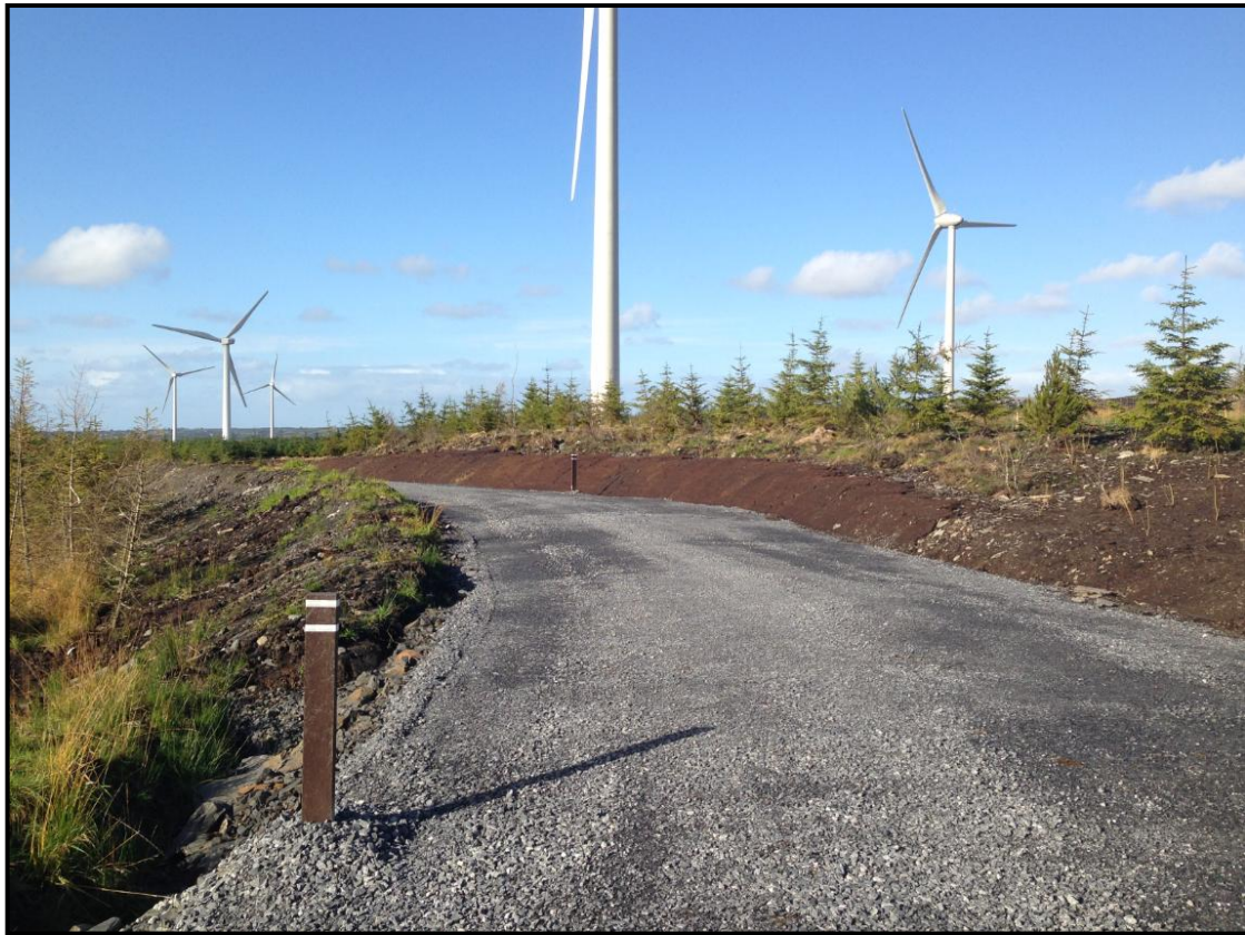
Figure 3-4: Typical Excavated Access Track
