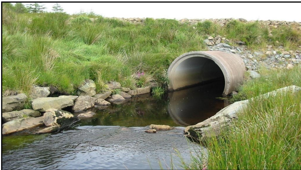
Figure 3-14: Typical Concrete Pipe Channel Crossing
