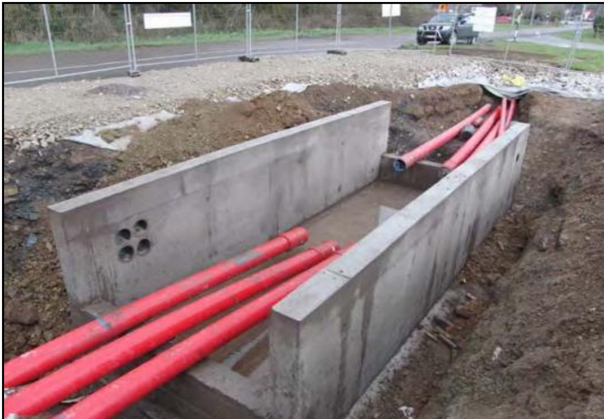
Figure 3-22: Typical Joint Bay Construction
