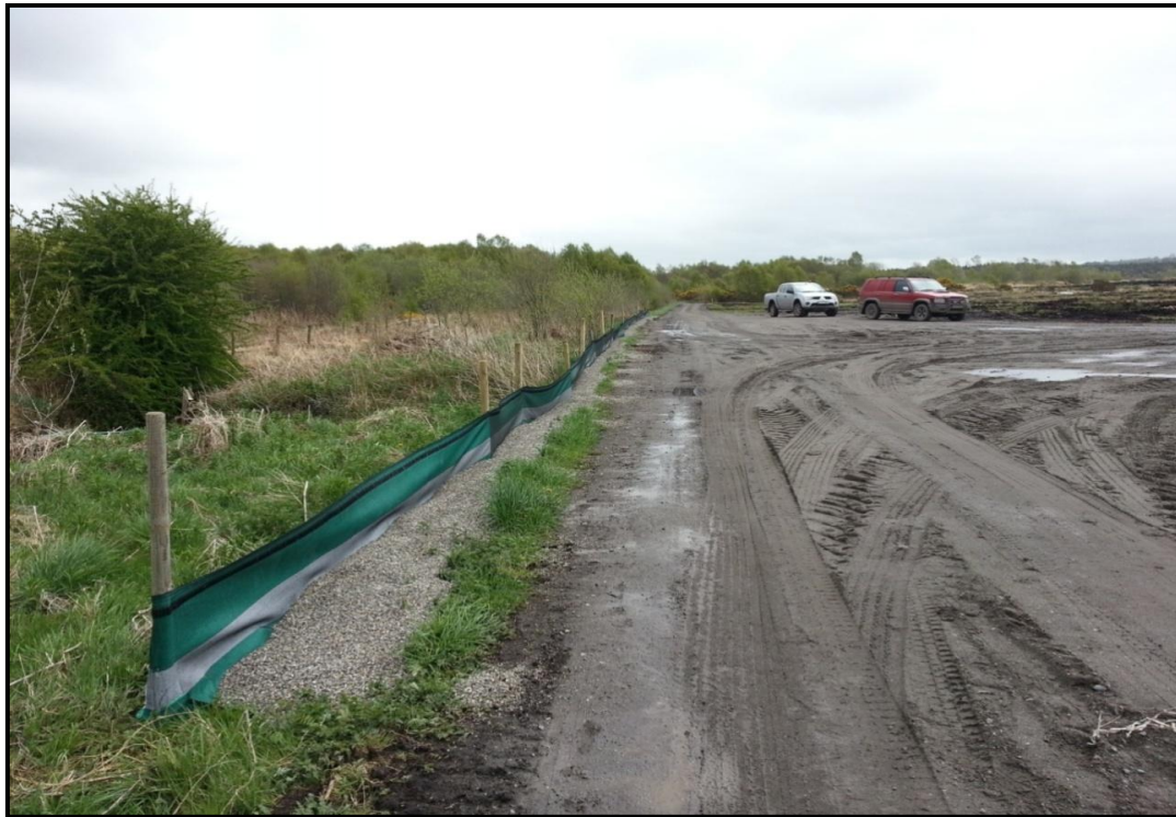
Figure 3-16: Silt Curtain Containment Along Tracks Near Watercourses
