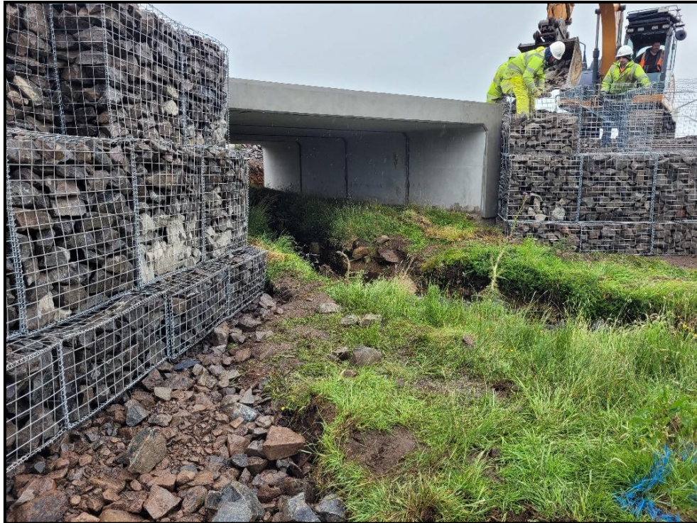
Figure 3-13: Typical Clear Span Pre-Cast Concrete Box Culvert Construction
