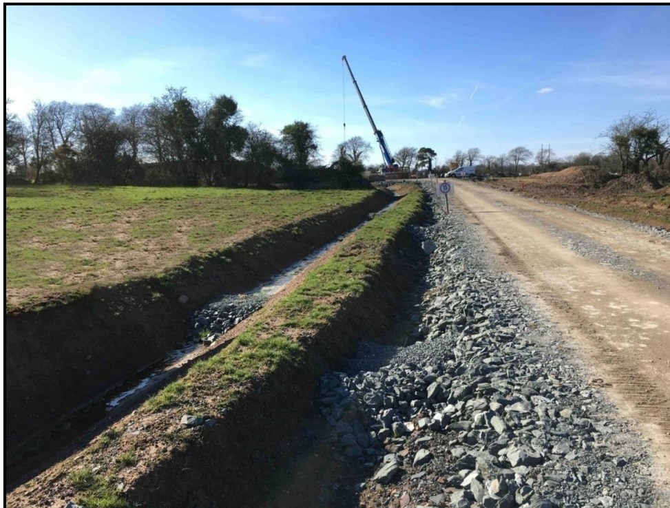
Figure 3-11: Separation of Clean and Dirty Water Drainage on A Wind Farm Site
